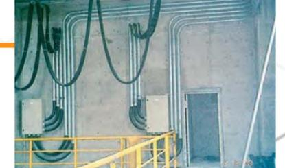
● 垃圾吊車縱行供電電纜 Long Travel Festooned Cables for Refuse Cranes
