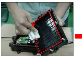
Clean the O-ring and the joint of the upper cover with alcohol.
