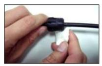
Clean fiber and the surface of fiber with alcohol.
